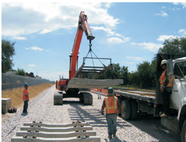
FrontRunner Track Construction
