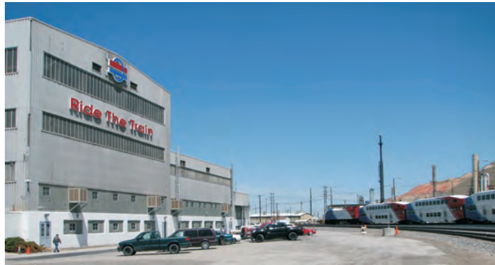
FrontRunner Service Facility
