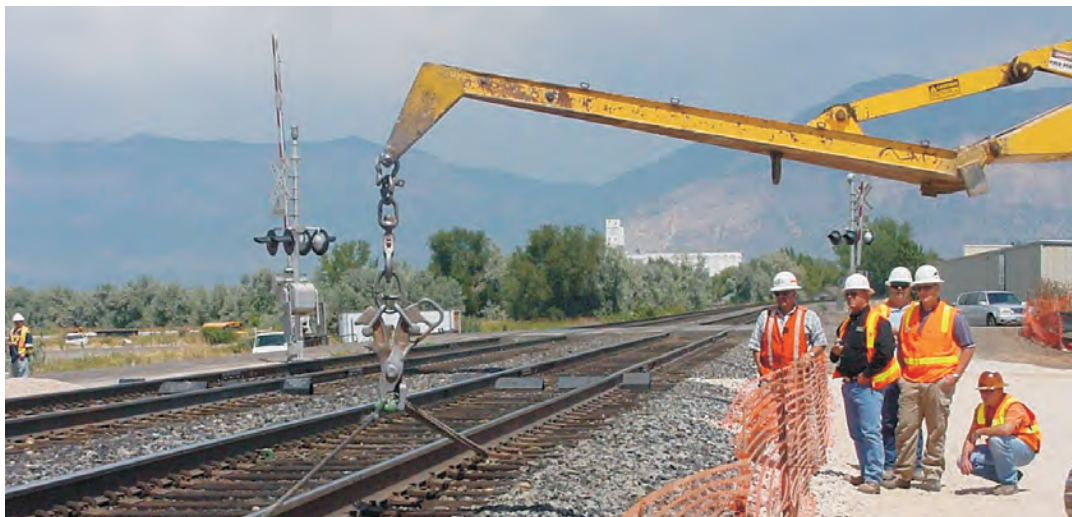
FrontRunner Track Construction
